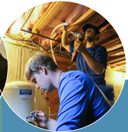
As a Technician-Assistant Apprentice , Jon Allen (foreground) works with Technician-Assistant Apprentice Tristan Wales from Roach Plumbing—an RWA Well Services Company.
