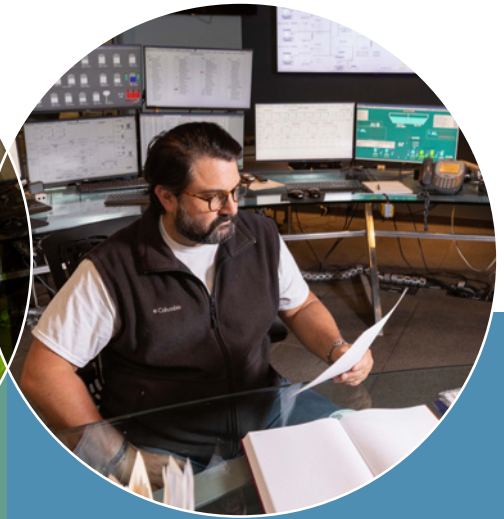
Mike Bova, Control Room Attendant , in the "nerve center" of the RWA's water distribution network. He, along with six other colleagues, monitors and manipulates the reliable operation of the RWA's distribution system 24/7/365.
