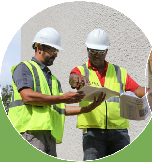
Brian Canterbury, Senior Project Engineer (left), and Orville Kelly, Manager of Design and Construction , review plans for the new one-million-gallon water tank in Derby that will provide storage to meet peak flows during maximum day demands and increase the amount of water available for emergencies.
