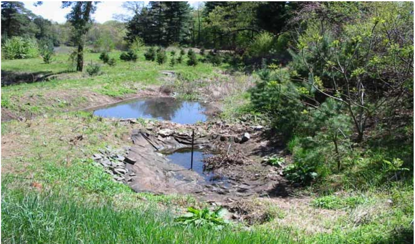
Figure 2. Treatment System No. 1 Forebay and Sedimentation Basin.
