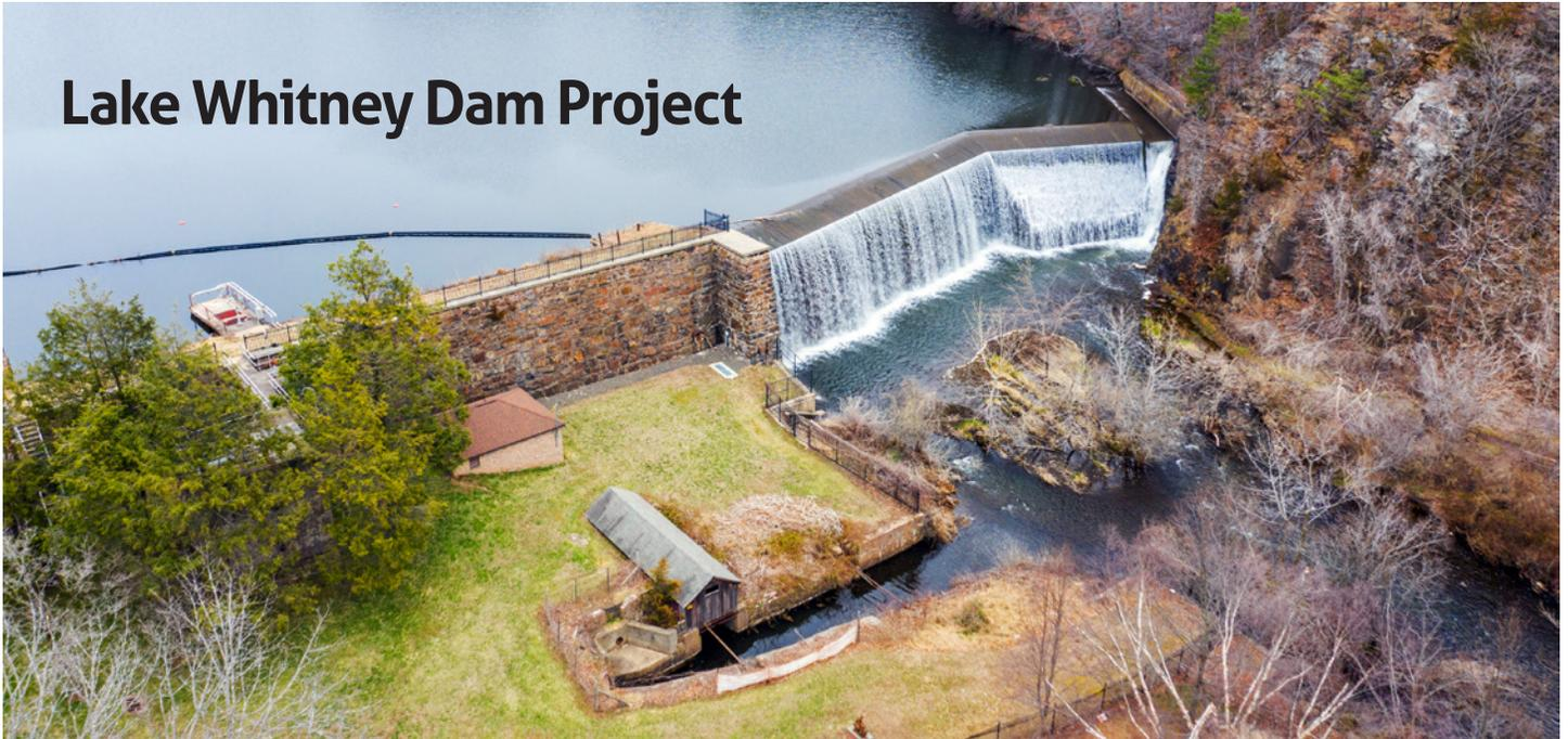
After over 160 years of service, it is time for the Lake Whitney Dam to be upgraded to meet future generations' needs. Lake Whitney Dam was completed in 1861 and was constructed with stone, rubble, mortar, concrete, and sand. While regular maintenance has been performed, the dam's structural aspects have remained largely unchanged since it was completed in 1861.
