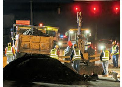
Water main breaks are serious and receive our immediate attention. When they occur, crews respond safely and quickly to make the repair and restore water service. Depending on the type of break, the water may be turned off. The RWA makes every effort to notify residents before this happens. A water main break usually takes four to six hours to repair.
