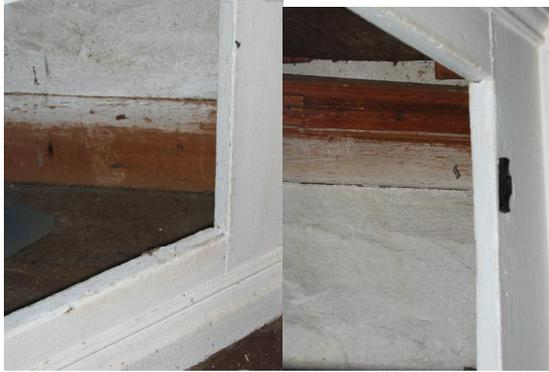
Figures 4 and 5 – Both the baseboard, left, and the chair rail, right, show that the corner cupboard has been in place since before the room received its first coat of paint.
