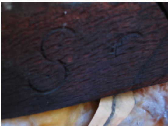
Figure 7 – The carpenter's marks on the brace between the southern plate and southeastern post.
