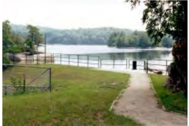
Walkway, Hand Railing
