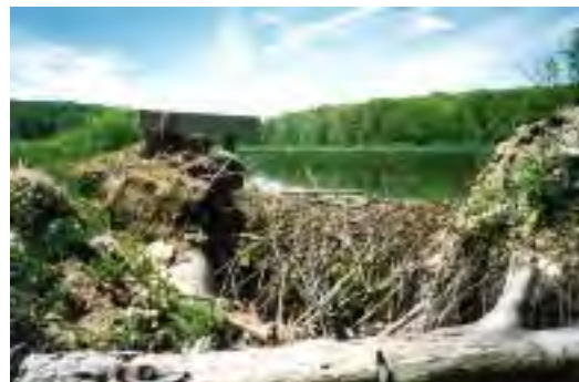
Beaver Dam in Spillway
