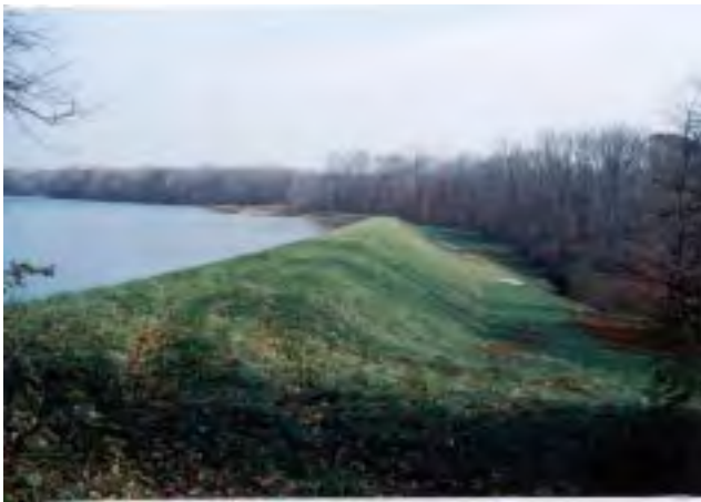
Well Maintained Embankment
