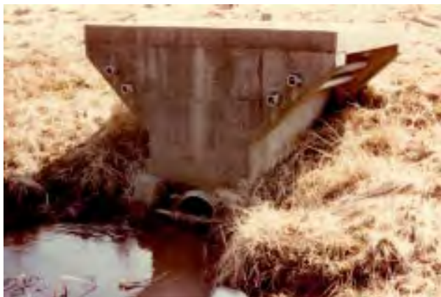
Concrete Intake Structure
