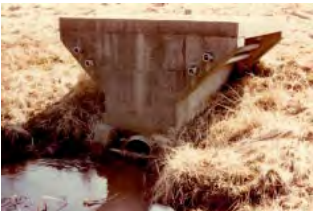
Concrete Intake Structure
