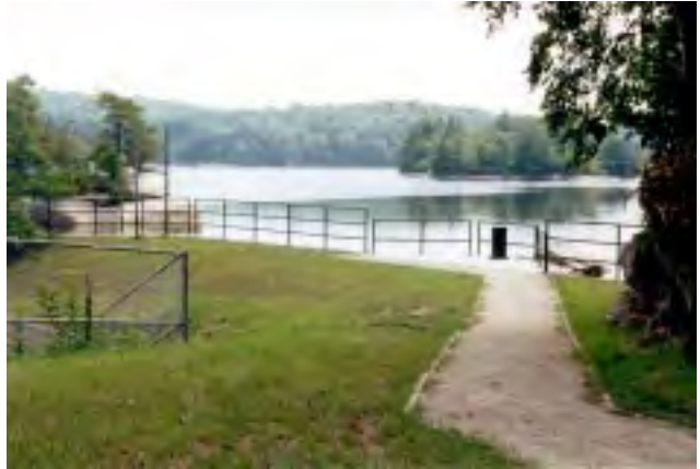
Walkway, Hand Railing
