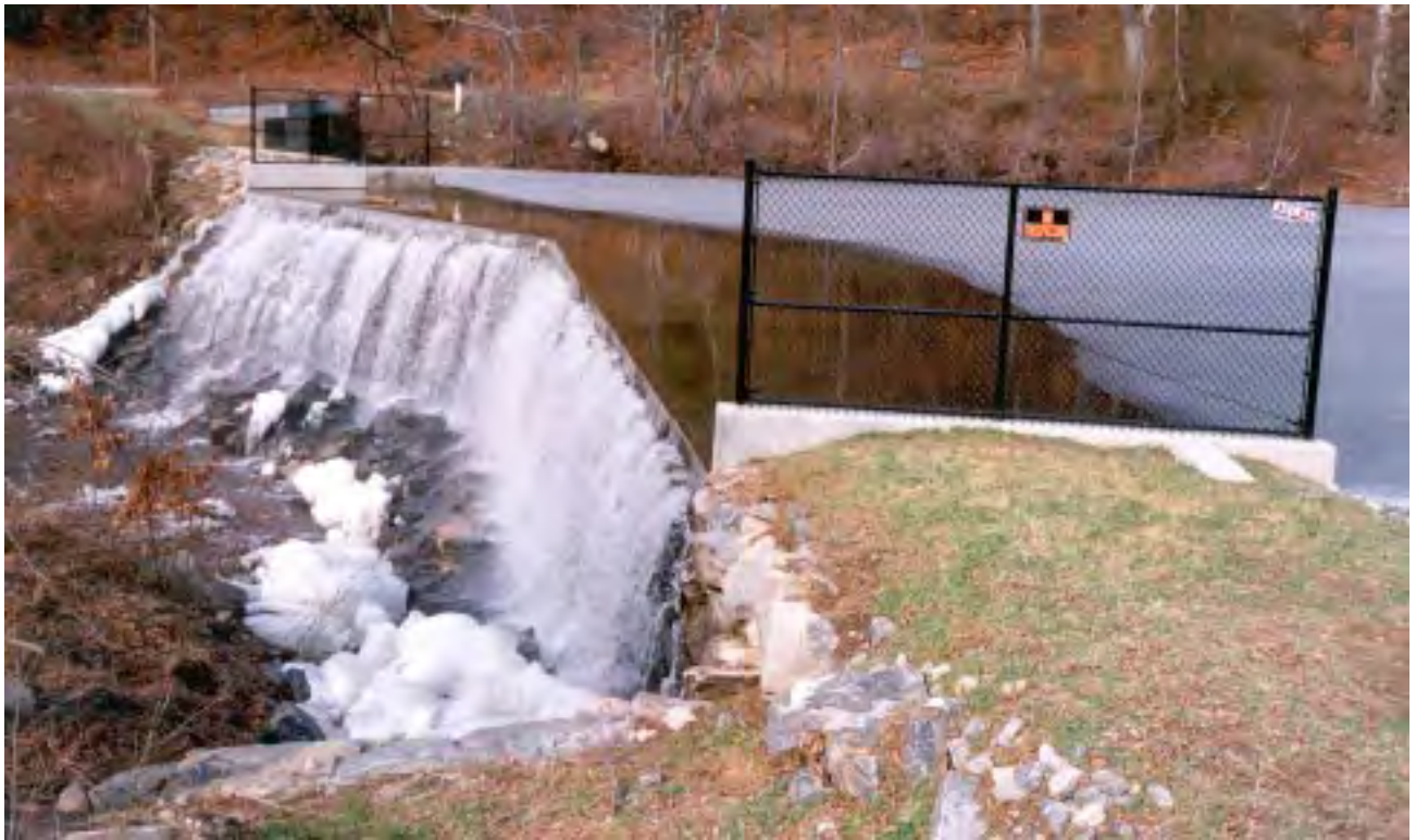
Fence and Signage
