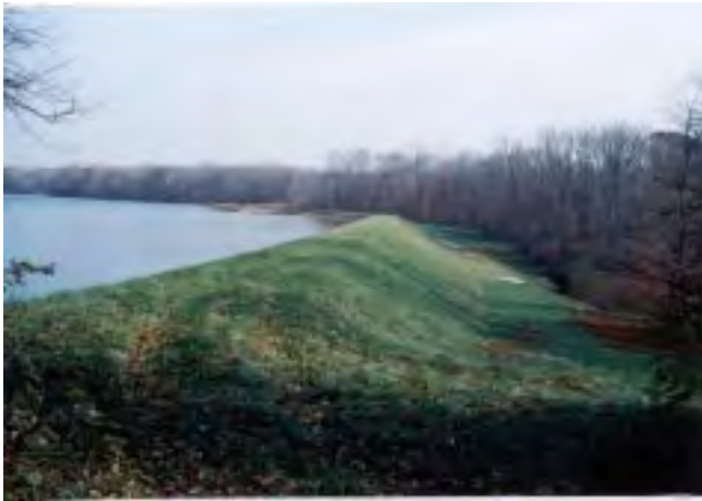
Well Maintained Embankment
