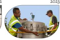
The RWA deployed the innovative NODES closed-loop water main cleaning equipment, which reduces discolored water concerns and preserves the water within our distribution system during flushing activities.
